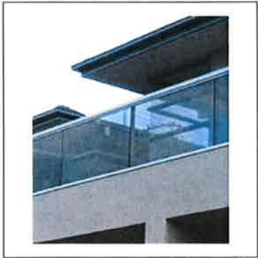
Clear/Tinted Glass Balustrade with Top Rail for Balcony
